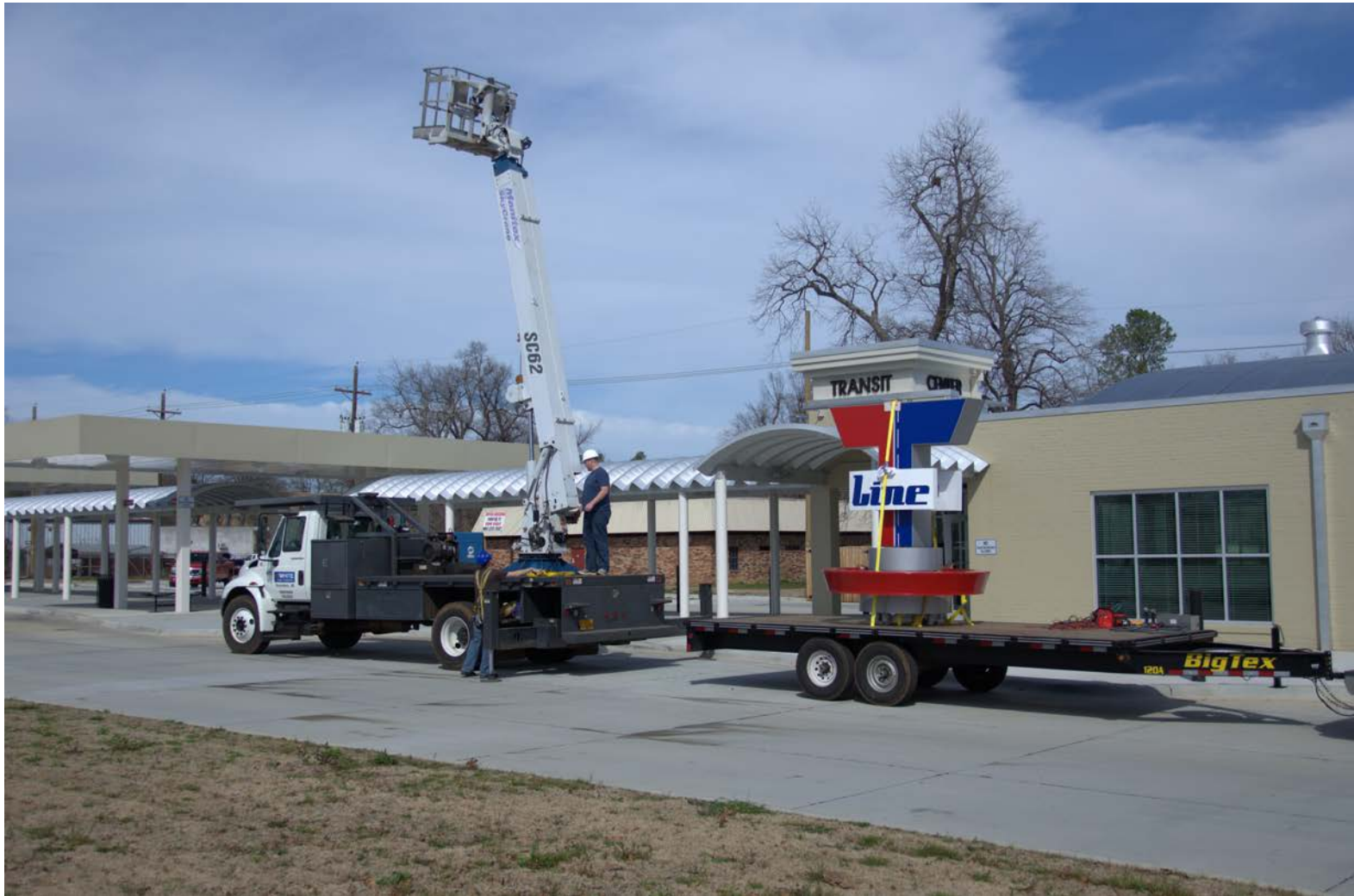
Preparing to install our New Revolving T-Line Sign
