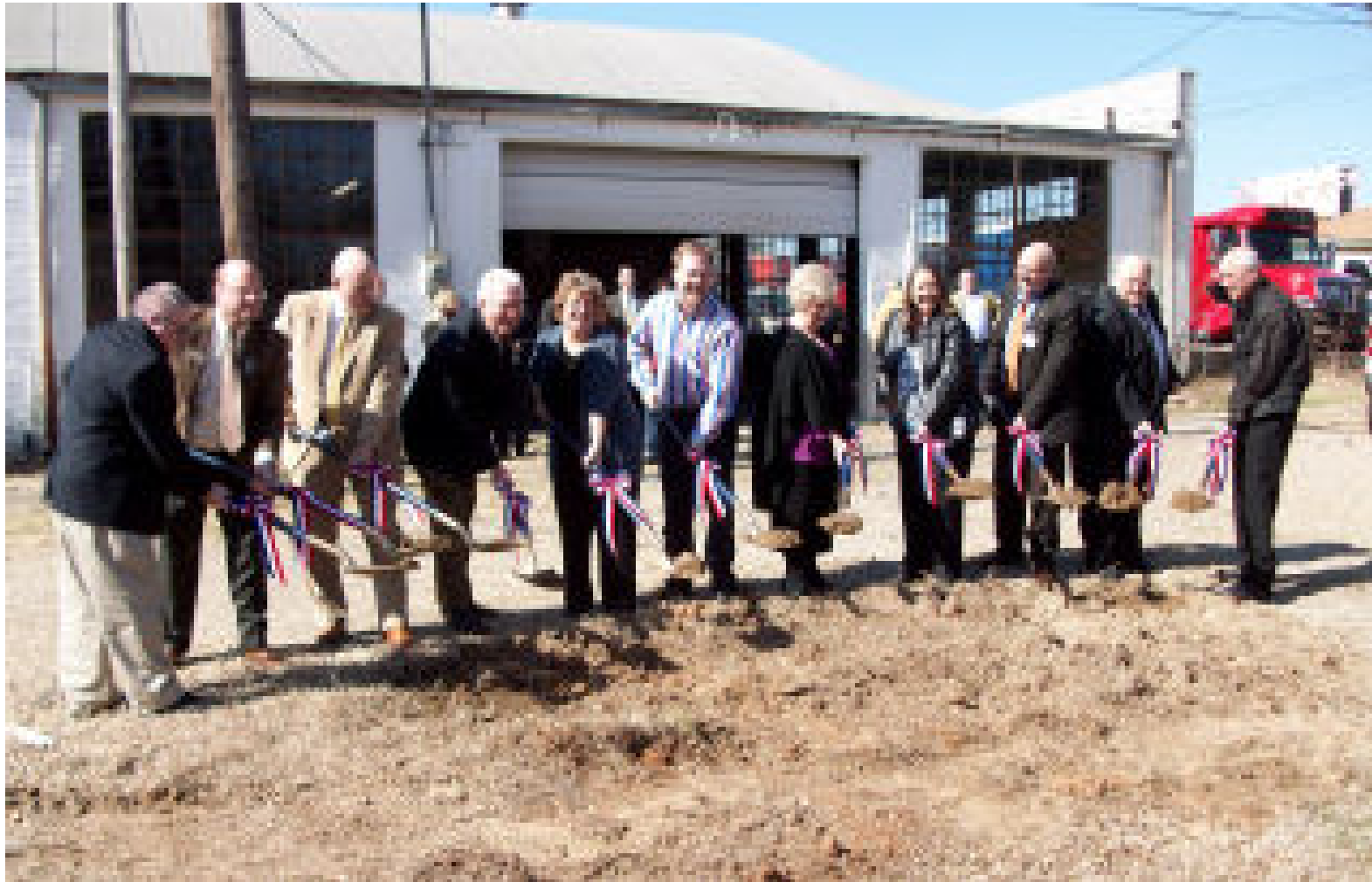
Ground Breaking Day for the future home of Texarkana Urban Transit District 1402 Texas Blvd. (2/18/10)
